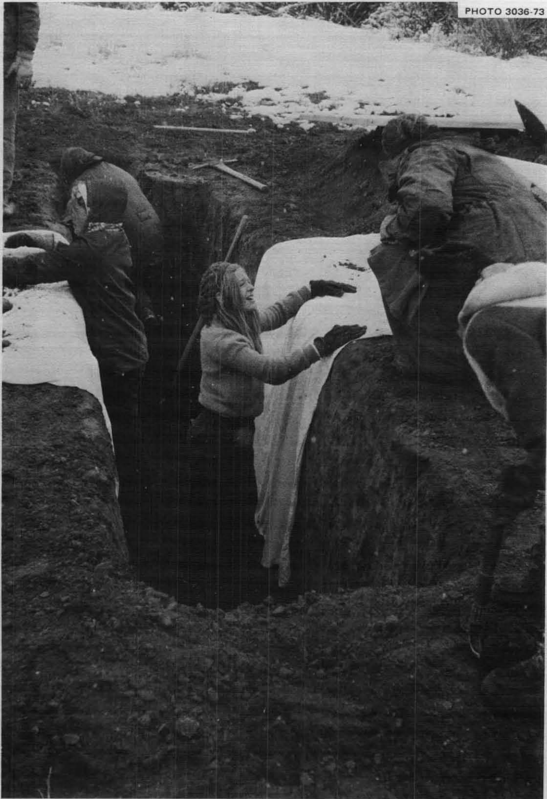
Fig. 2.8. Placing bedsheet coverings on the 4\frac{1}{2} -ft-high trench walls. Such coverings make the trench cleaner, warmer, and easier to illuminate.
